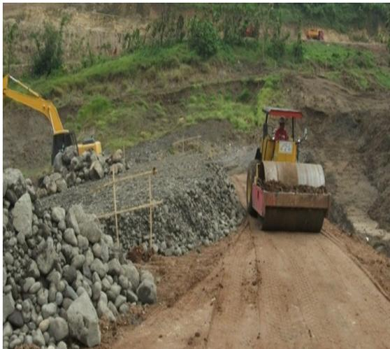
**Gambar 6.** Pemasangan Timbunan *Saddle Dam*
