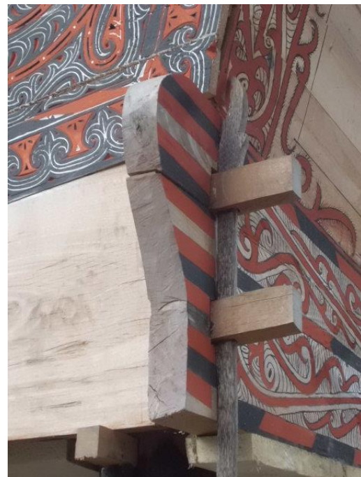
Figure 6. Tectonics of a peg hole in the wall (Source: research documentation 2018)
